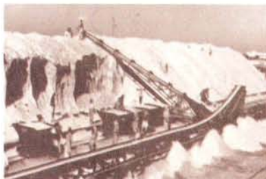
Mechanical stacking of washed salt.
