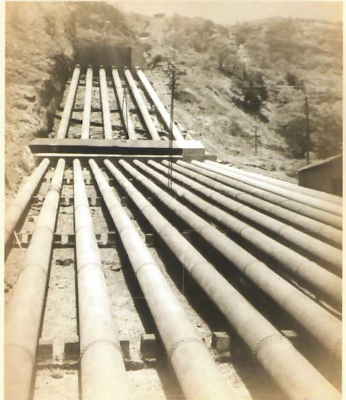
Penstocks carry water downhill from the lakes to the generating stations.
